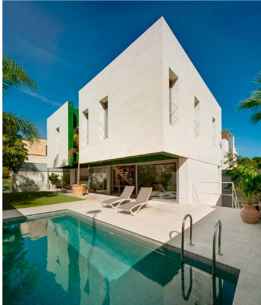
Private House, Alicante, Spain .
